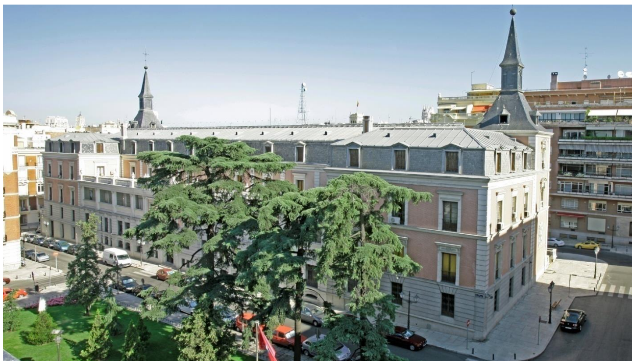
Main south façade.
