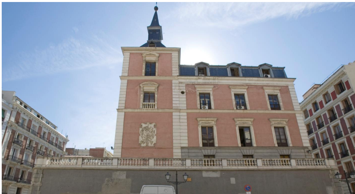
West side façade.
