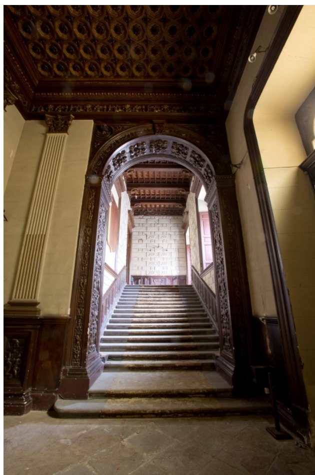
Escalera de Honor (Stairway of Honour). Level 0.
