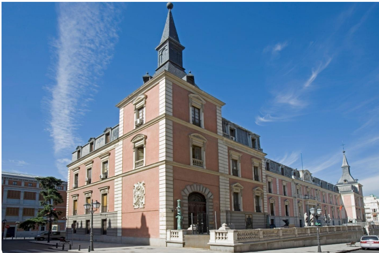
East side façade and main north façade.
