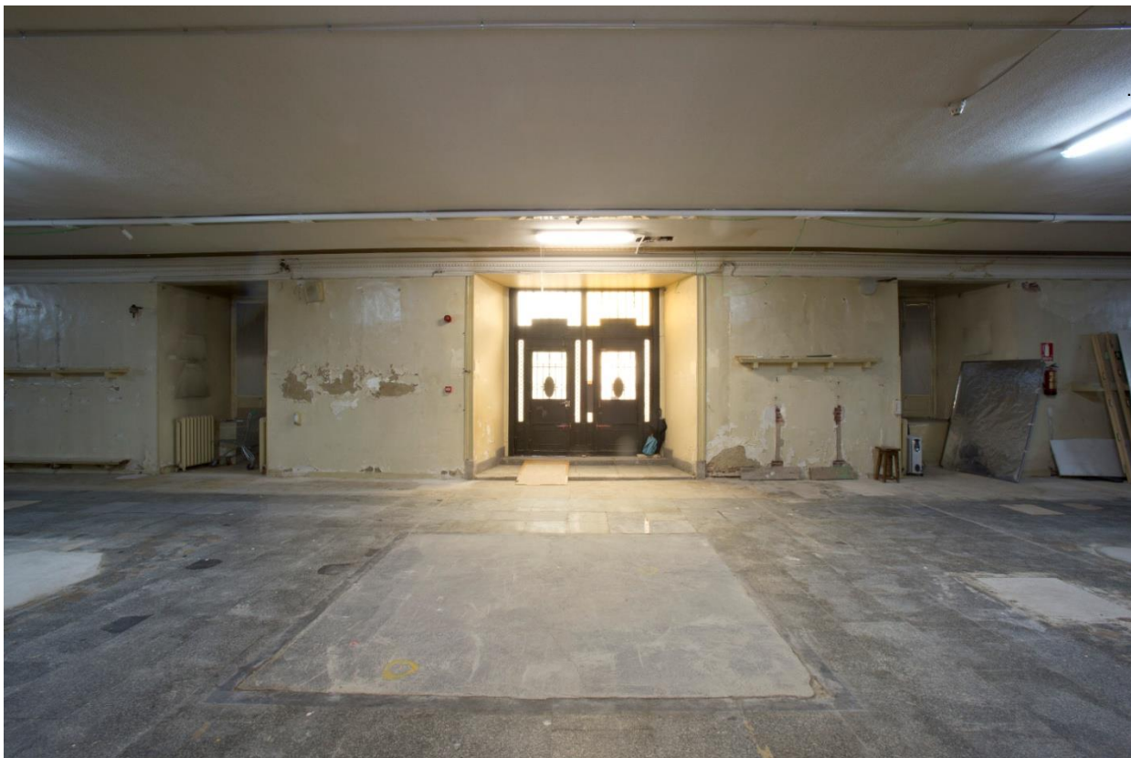
Sala de Artillería (Artillery Hall). Northern central access. Level 0.
