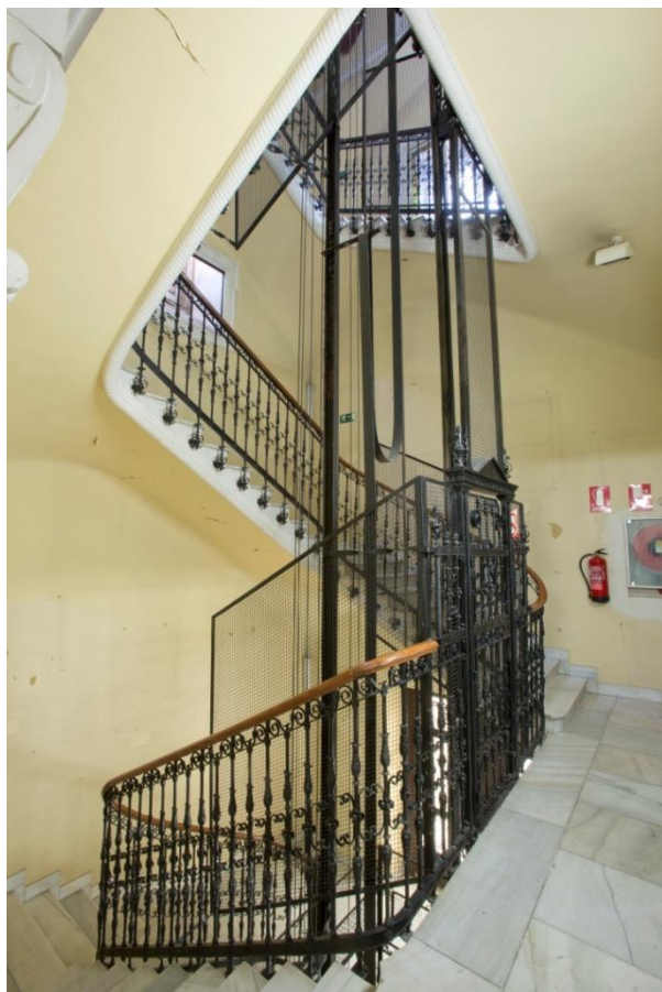
Northwest vertical connecting core.
