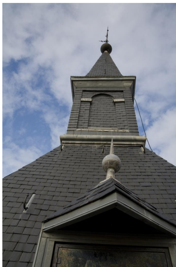
West tower. Roof detail.
