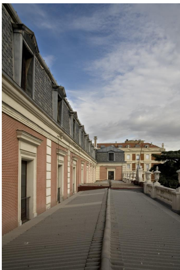
South façade. Second floor roof.
